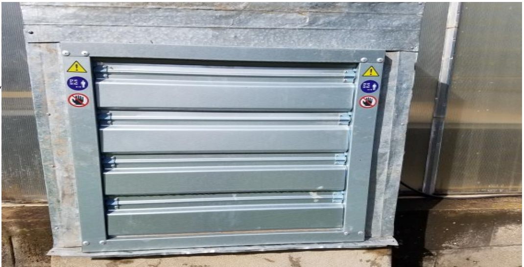
Fig.42. New greenhouse fans purchased and the motors of old fans rewired
