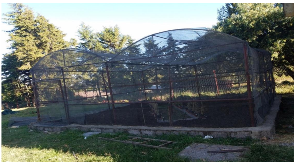
Fig.32. Aditonal Lath-house constructed at KARC
